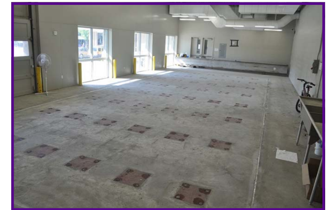
Completed strong floor showing 50-kip anchorage points
