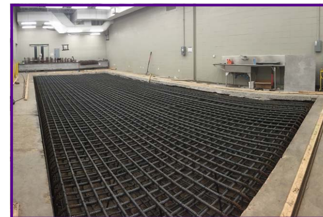
Heavy steel reinforcement in 4-ft thick strong floor
